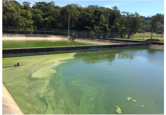
This Sludge lagoon allows the sludge to settle. Due to the large ratio of water, it is returned to the head of the work to be processed again. Due to the small population this treatment plant caters for, this tank only needs to be emptied every 5 years.
