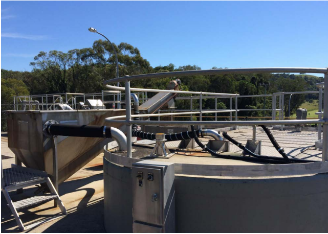
This 'Grit Arrester' creates a vortex by pumping air into the water which lifts the sand and grit off the bottom.
