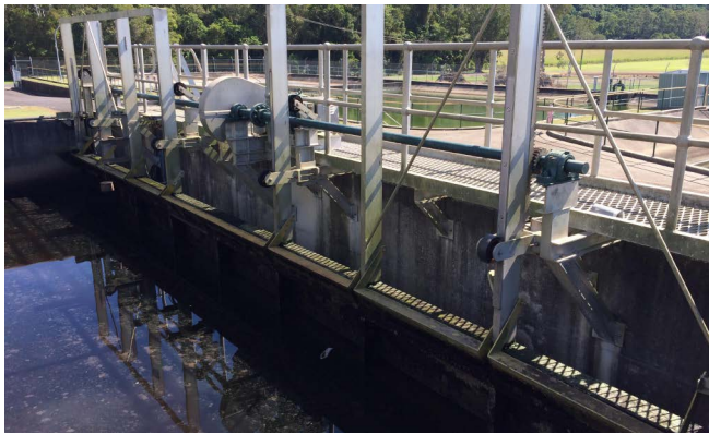
This 'Extended Aeration Tank' adds oxygen to the water which allows the bugs to eliminate the ammonia and nitrogen. The sludge which contains the microorganisms settles on the bottom. This weir board lowers enough to decant the clear water into a tertiary pond.
