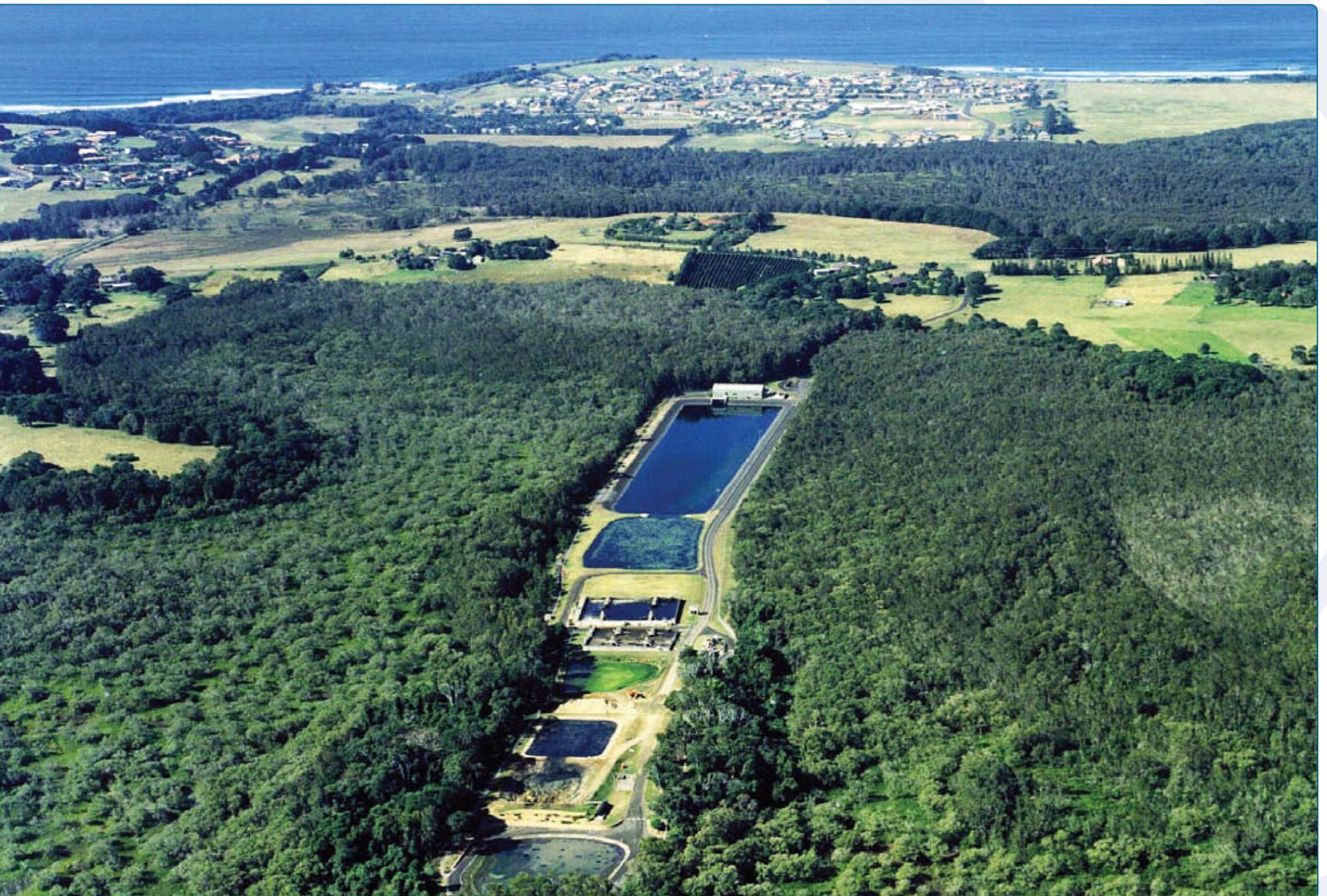
Lennox Head Wastewater Treatment Plant
