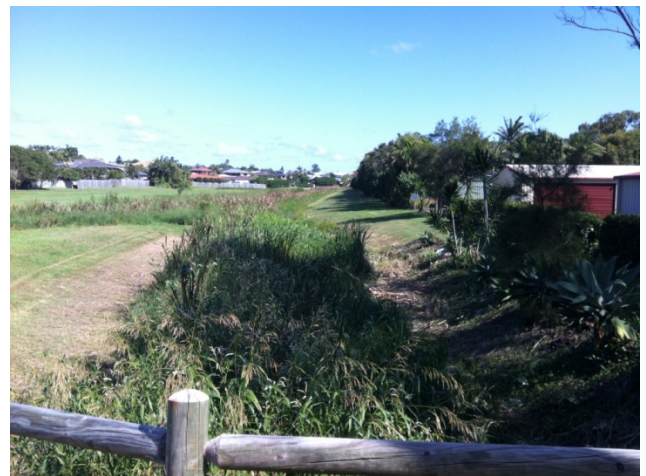
Photo 8: Drain at Skennars Head behind Headlands Leisure Centre overgrown with Phragmites
