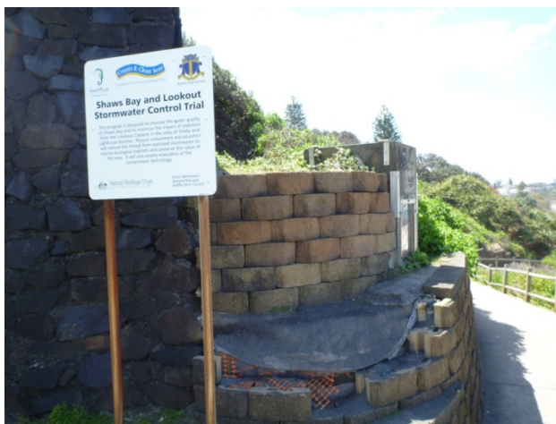
Photo 10: Shaws Bay Stormwater Control Trial
