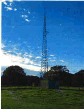
Figure 3 – Existing Northern Communications Facility
