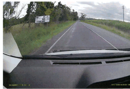
2. Ross Lane Westbound East of North Creek
