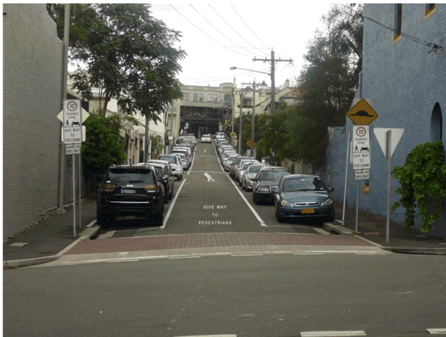
Figure 2. Photo and diagram of a Category 2 shared zone showing regulatory signage, entry treatments, traffic calming, parking provision, and typical layout. The photo may have been modified to demonstrate essential elements.
