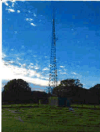
Figure 3 – Existing Northern Communications Facility
