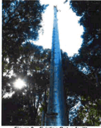
Figure 2 – Existing Optus facility
