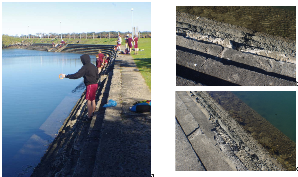
Figure 18: Training wall concrete steps
