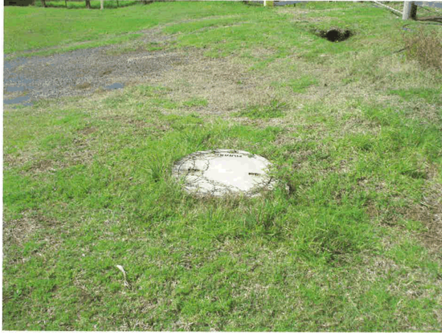
Photo 7. Sewerage Pit Cover Bottom Access Road Next To Easement
