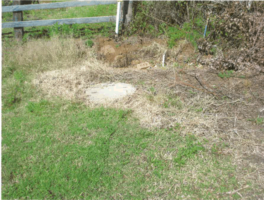
Photo 3. Storm Water Access Pit Cover Top Lot 1. Beside Easement
