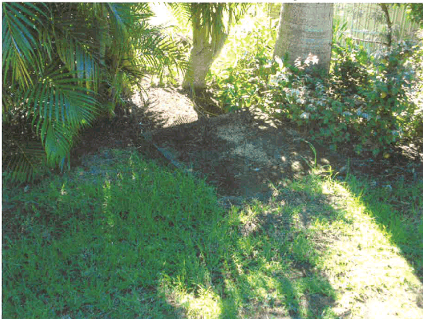
Photo 6. Storm Water Access Pit Cover Top Lot 1. Beside Our Land. This is the Site of the Planned Grilled Pit to Catch All the Diverted Storm Water.
