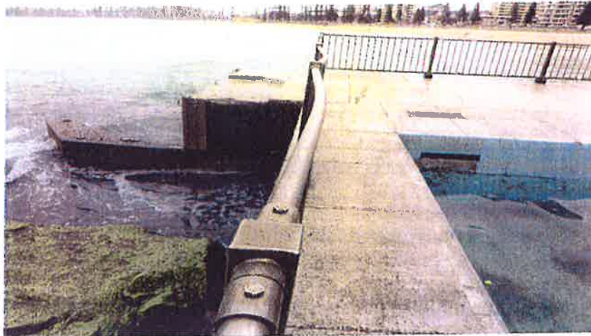
LARGE OUTLET 4 – 5 METRES WIDE (Southern Side)
