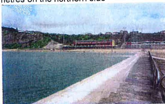
WALL 3 METRES WIDE NORTHERN SIDE
