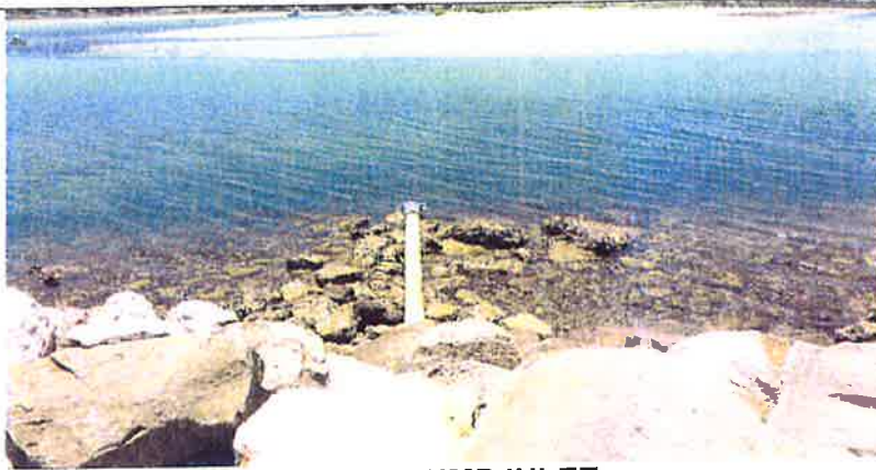
RIVER PUMP INLET
