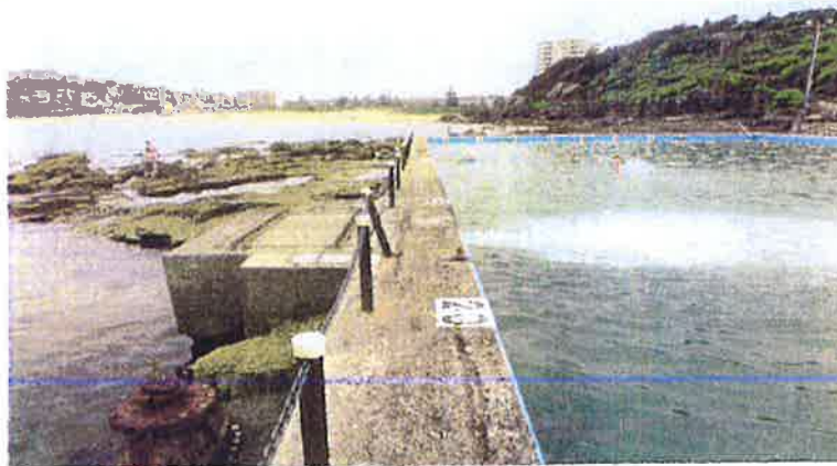
PUMP HOUSE AND INLET
