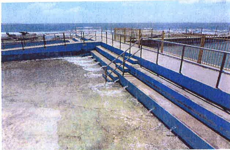
WADING POOL BEING FILLED AFTER CLEANING NOTE: THE EXTENSIVE USE OF FENCING AND HAND RAILS
