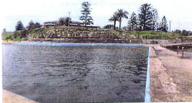
MAJOR REFURBISHMENT 3 YEARS AGO
