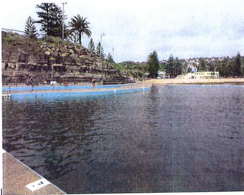
COLLARROY POOL IS WELL USED AND WELL MAINTAINED
