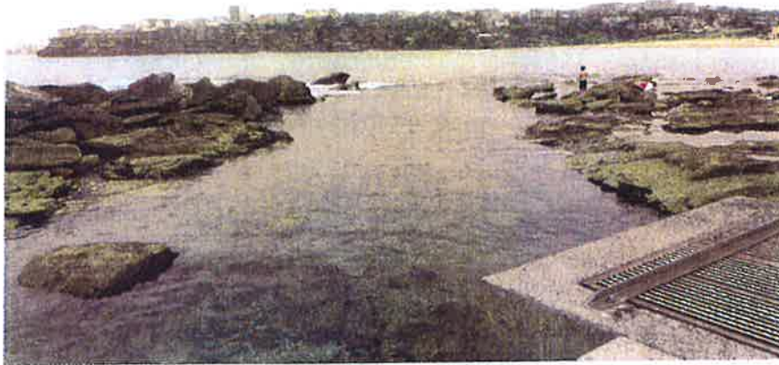
PUMP INLET TRENCH (Planned To Deepen)
