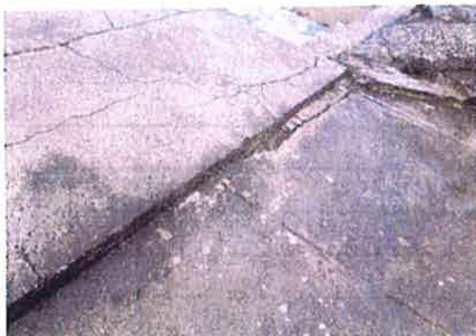
CRACKING/TRIP HAZARDS
