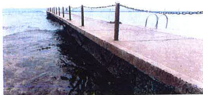
CANTILEVERED USING STAINLESS STEEL SUPPORTS
