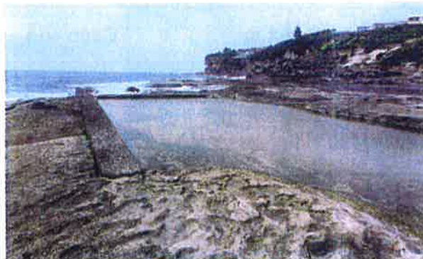
SHALLOW LOW WALL POOL EASTERN SIDE
