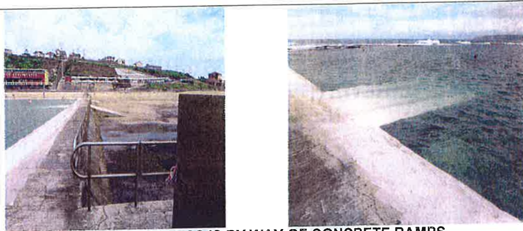
POOL ACCESS IS BY WAY OF CONCRETE RAMPS
