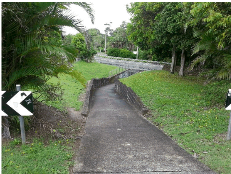
Photo 4 – Pedestrian access way at the southern end of Greenwood Place leading to Byron Bay Road underpass
