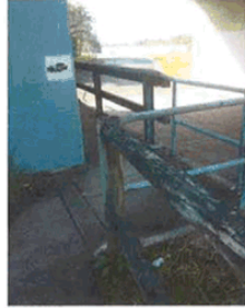
Photo 3. Dogleg. Looking east.
