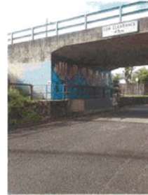
Photo 6. The footpath under the bridge
