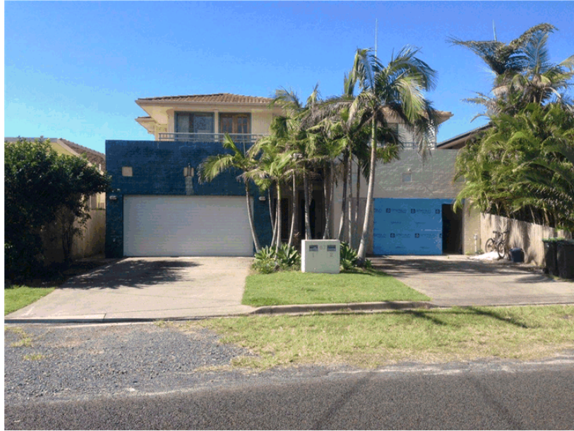
DA 2015/204 photos of Units 1 and 2/67 Stewart Street, Lennox Head
