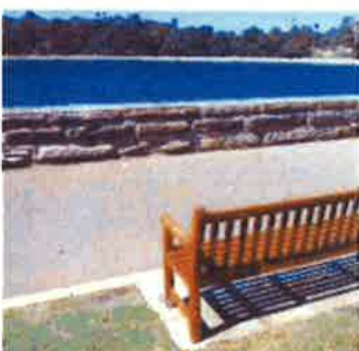
Botanical Gardens, Sydney- stone wall [note no skateboard damage on capping]
