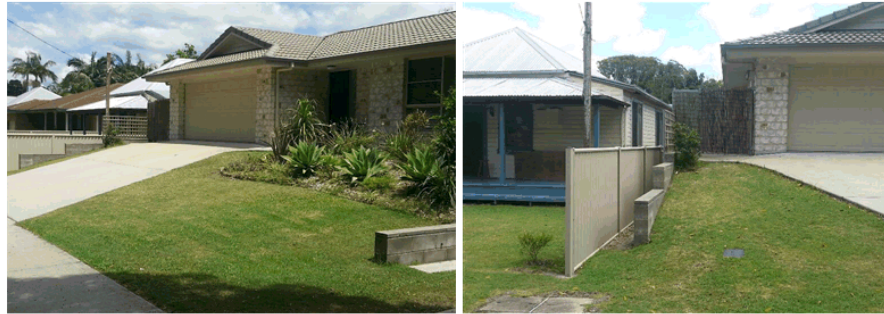
Photos 4 and 5 show a dwelling constructed in Richmond Street, Wardell in 2009
