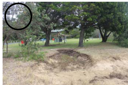
erosion at the foreshore
