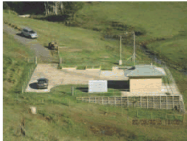
Lot 9 - actual view over pump station
