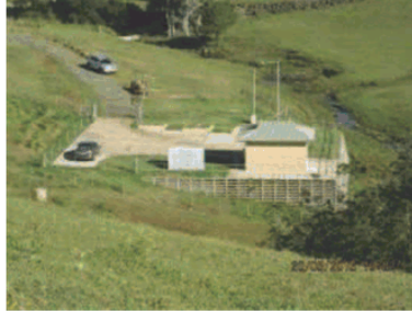
Lot 8 south sector - view over pump station
