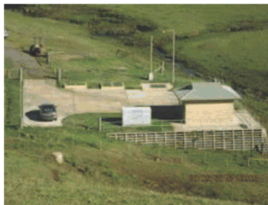
Lot 10 - actual view over pump station
