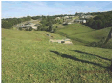
Lot 9 - distant view over pump station
