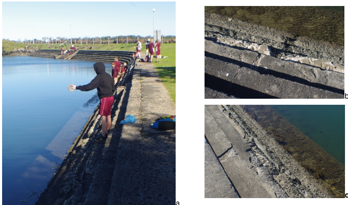
Figure 20: Training wall concrete steps
