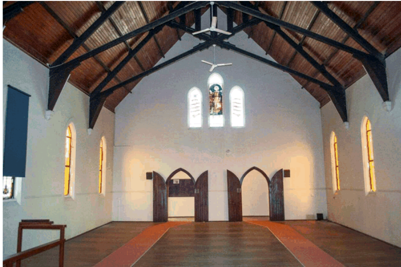
Above: Image shows the exposed scissor truss, pine lining, decorative windows located on the church's front façade, and the twin Gothic arch doorways that lead into the nave.
