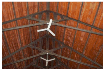
Above: Image shows the exposed scissor truss, pine lining, decorative windows located on the church's front façade, and the twin Gothic arch doorways that lead into the nave.
