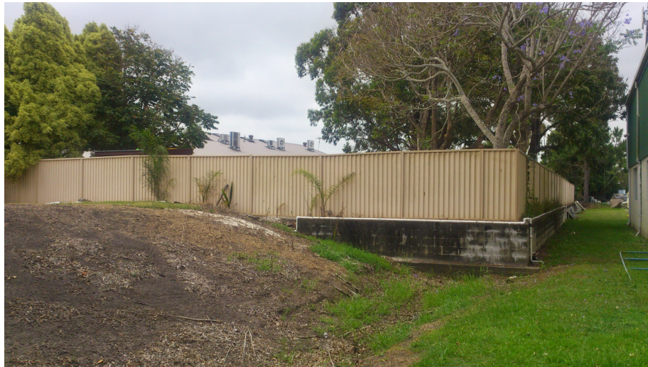
Buffer looking west from Sunset Avenue
