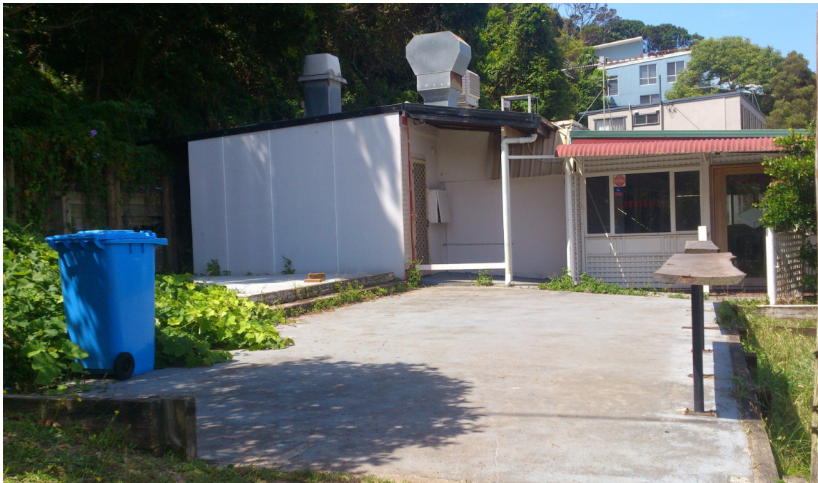
Site photo 18 – Compton Drive restaurant site lease area
