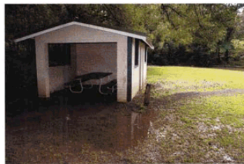
Change Rooms shed after May 2015 flood
