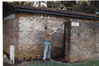
Lions Club doing maintenance on Toilet Block, 1990
