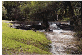
Bulwinkel Weir in flood, May 2015
