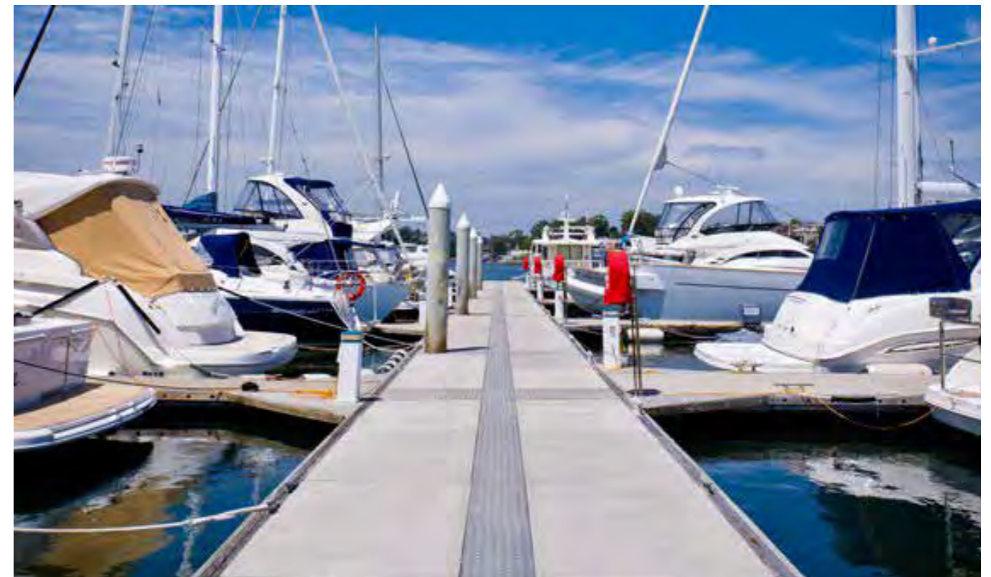
New marina infrastructure will greatly enhance the value and operation of the harbour as a key boating facility
