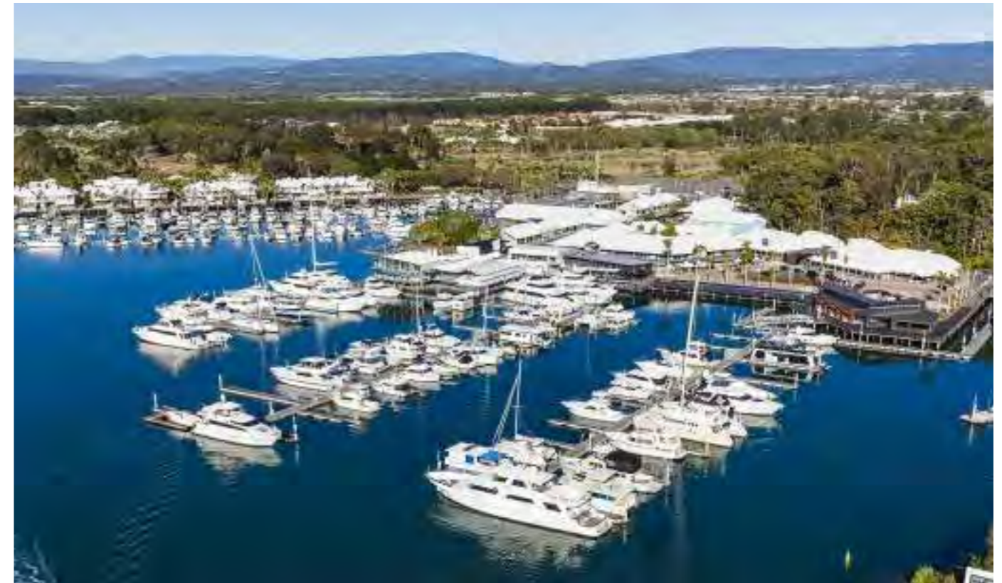
The new marina will allow significant additional berths and provide much-needed capacity for visiting craft
