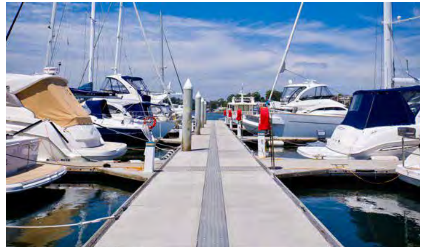
New marina infrastructure will greatly enhance the value and operation of the harbour as a key boating facility
