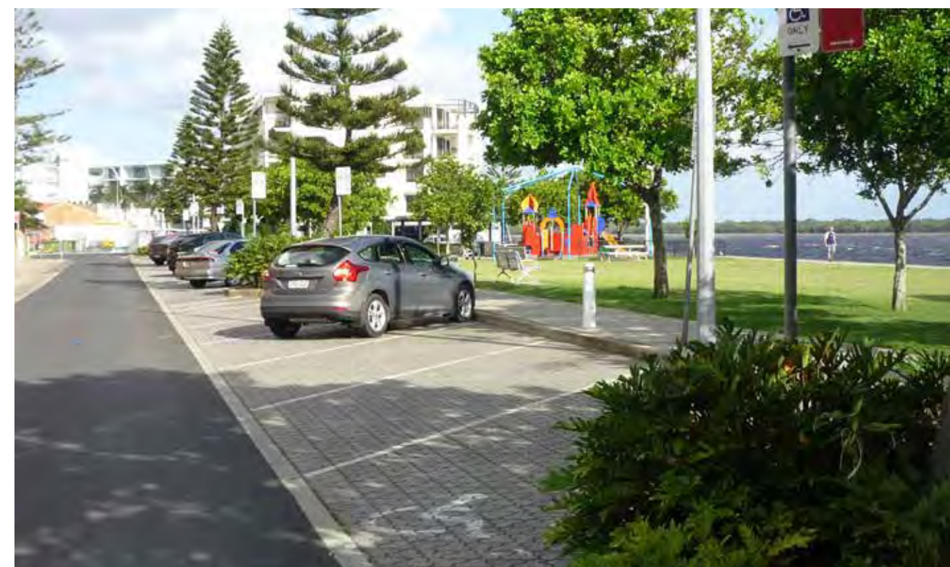
A new one-way system with angled parking will greatly improve traffic management in Regatta Avenue
