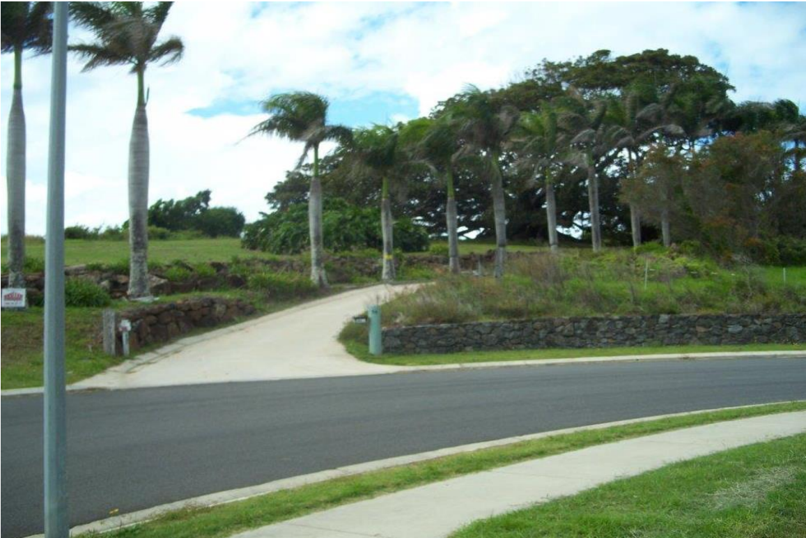
Existing entrance driveway from Blue Seas Parade located in north-eastern most section of site.
