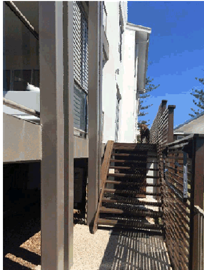
Northern wall and patio showing natural sunlight that will be lost resulting from the proposed encroachment.
