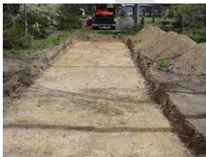
Wick Trench Installation Photos
