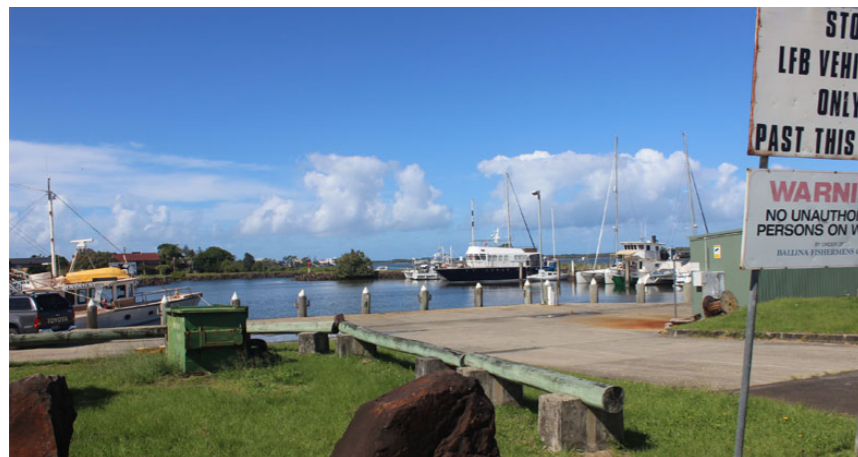
O existing concrete wharf at the harbour
