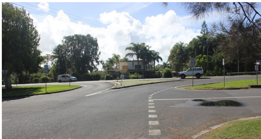
D River Street and Boatharbour Road intersection
