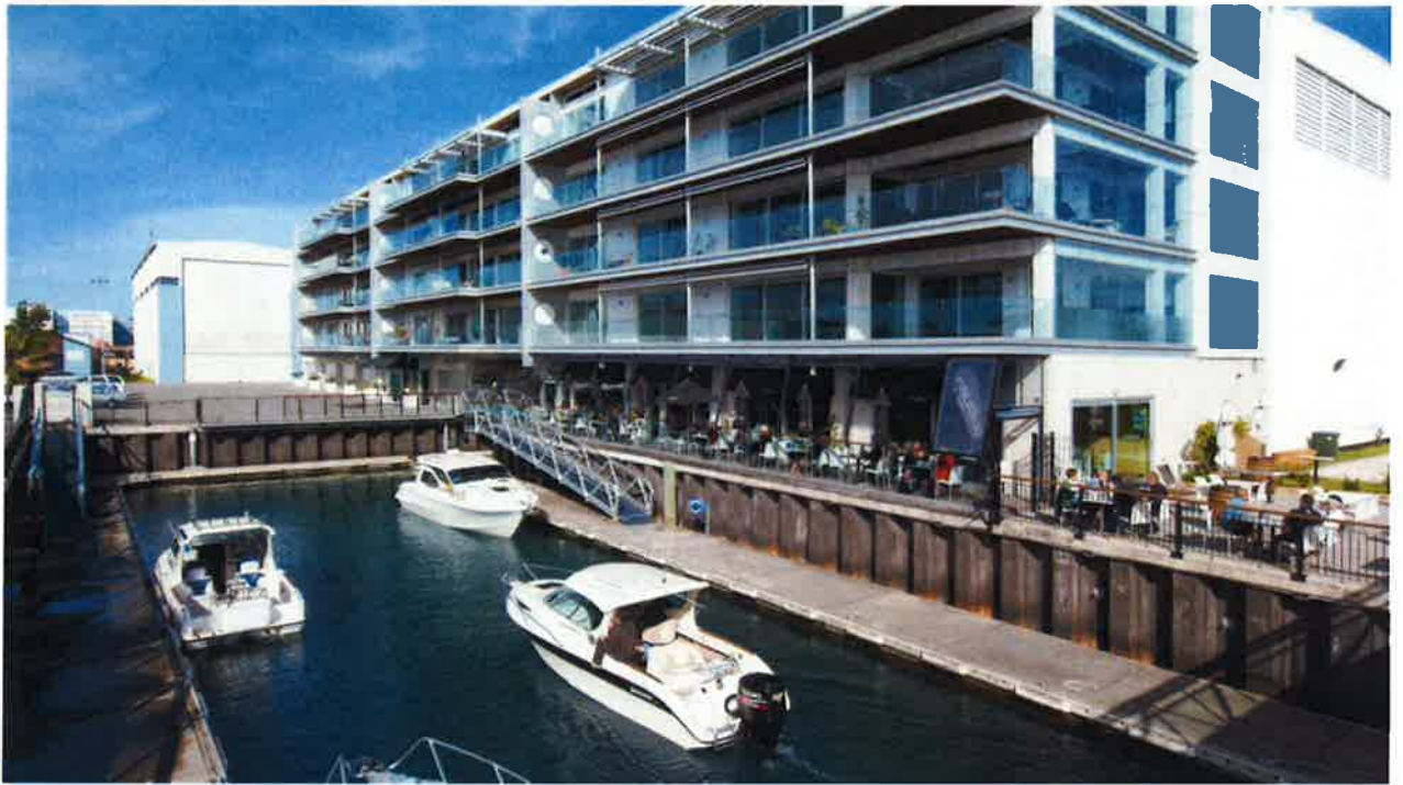
PHOTO SHOWING RESTAURANT & RETAIL SHOPS PLUS 4 LEVELS OF APARTMENTS
