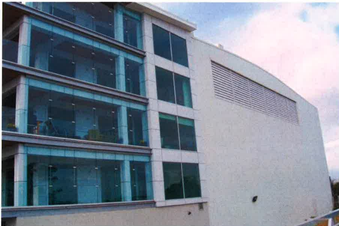
NORTH-WESTERN FAÇADE SHOWING APARTMENTS AND DRY STACK SECTIONS
