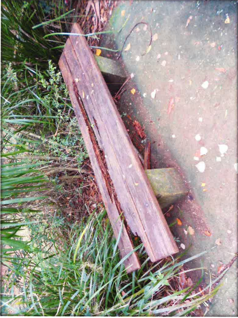
Figure 7: Replace rotten top on existing seat
