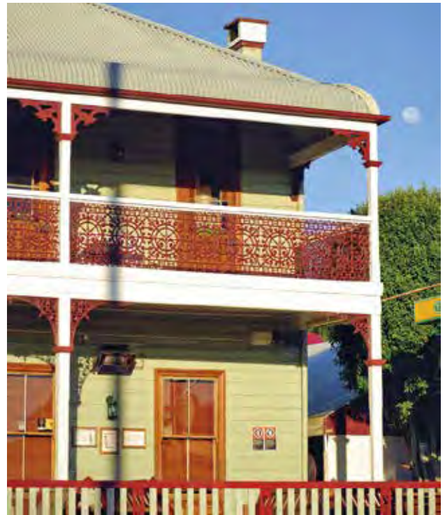
Federal Hotel, Main Street, Alstonville
