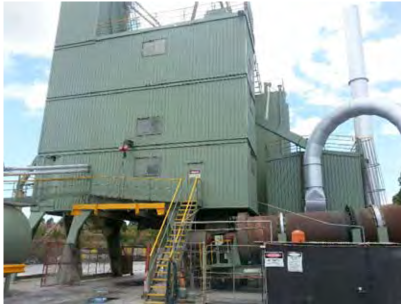
Asphalt plant within Tuckombil Quarry Site
