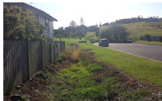
Photo H - Hutley Drive and drain
