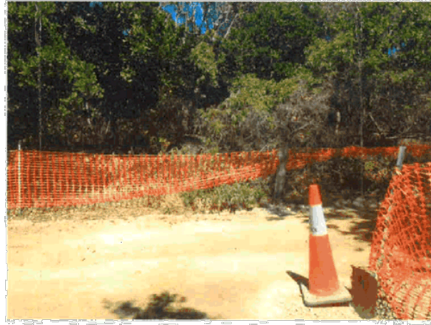
Option 1 and 3: 4WD access crossing location at CRP (view to west towards The Coast Road)
