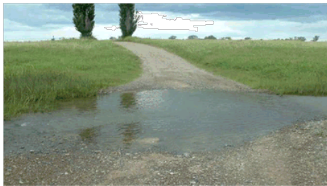
Figure 3: Fish-passage friendly water-crossing
