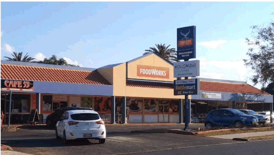
Photo No. 18: Location 2 PM: Foodworks Shopping Centre, view to the South
