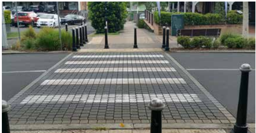
Main Street beautification works completed in 2010-2011
