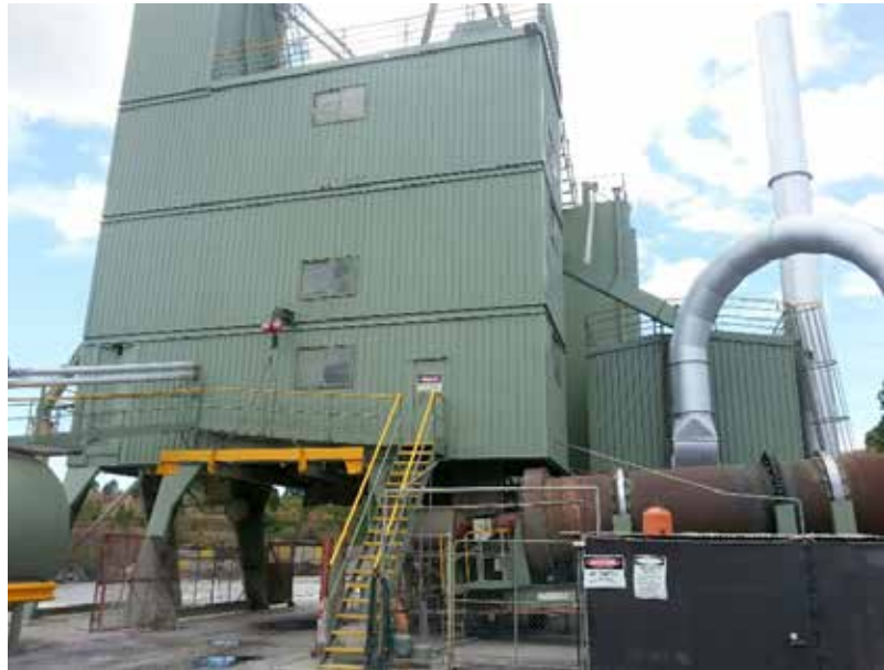
Asphalt plant within Tuckombil Quarry Site
