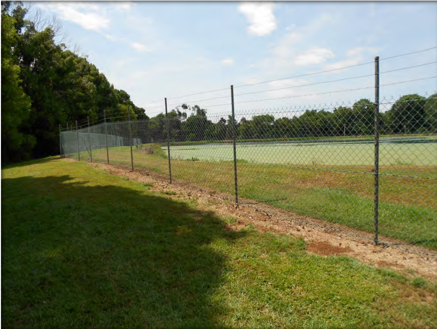
Figure 18: Security mesh fencing with barbed wire to deter trespass
