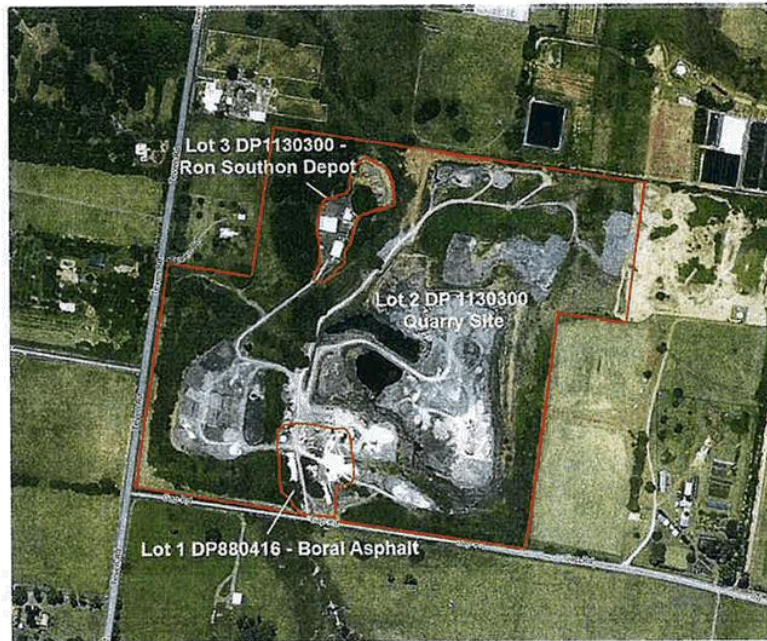
Figure 2: Showing Quarry site and 2 associated businesses located within the Quarry site – Ron Southon Pty Ltd and Boral Asphalt.
