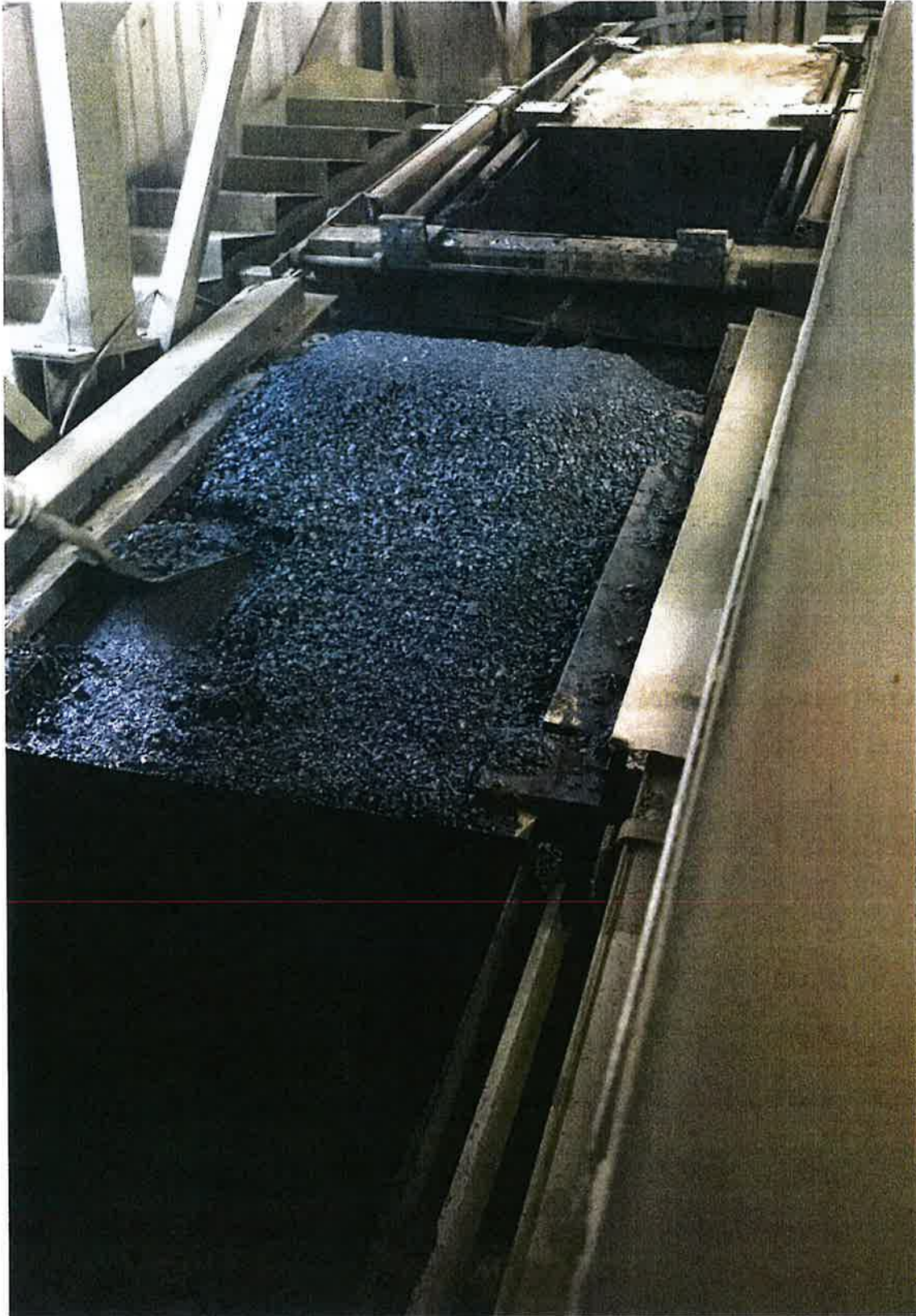
Figure 3-6 Hot asphalt storage bin, with the skip conveyor approaching and preparing to be sampled
