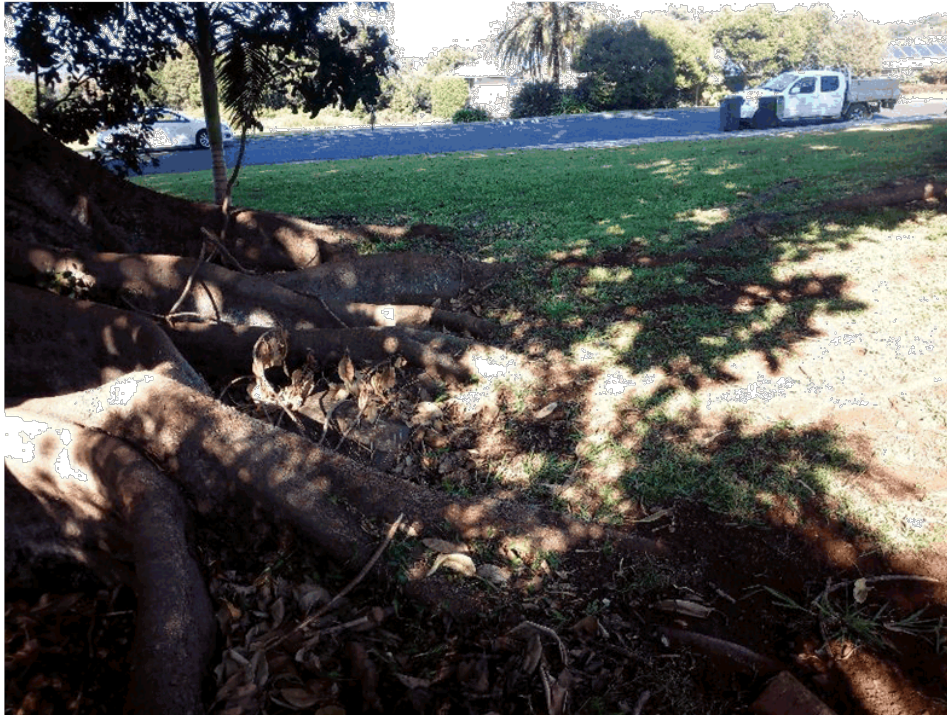
150749 2015-08-19 V1 Ballina SC Subsidence-Tree Root Damage
