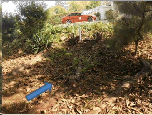
20: Tree roots running towards the driveway
