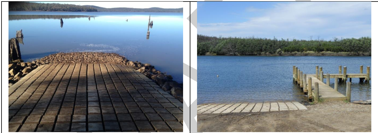
Figure 1. Concrete Flexmat™ (or comparable product) ramp at Tooms Lake, Tasmania (left) and Upper Scamander River, Tasmania (right).
