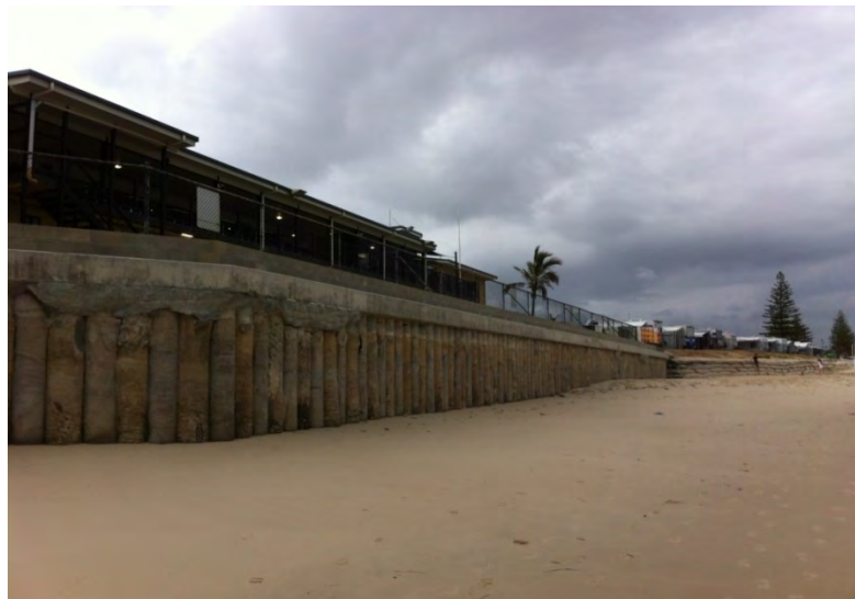
Figure 9-6 Secant Pile Seawall at Kingscliff Beach
