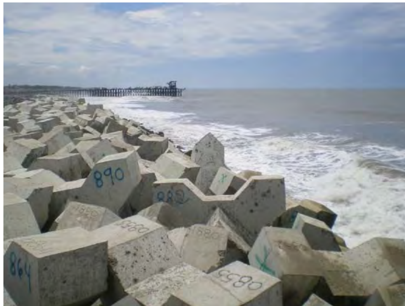
Figure 9-4 Randomly-Place Concrete Revetment (Photo courtesy Xbloc)
