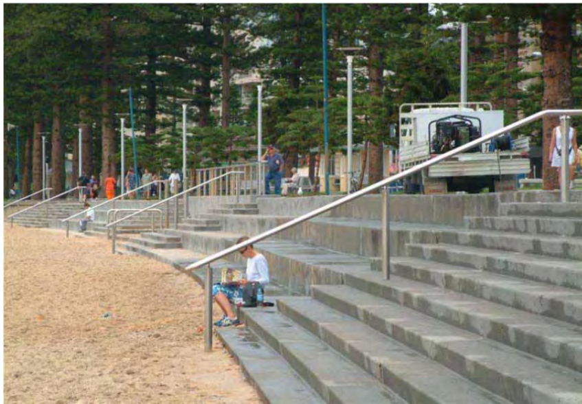
Figure 9-5 Stepped Seawall at Manly Beach, NSW (Photo from WRL, 2012)
