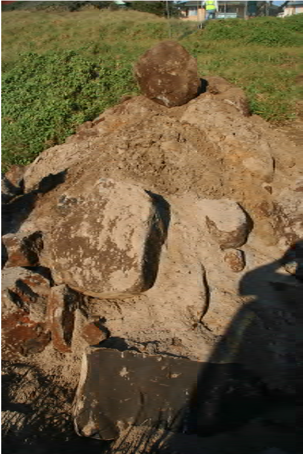
Figure 4-12 Exposed Rocks in Existing Seawall
