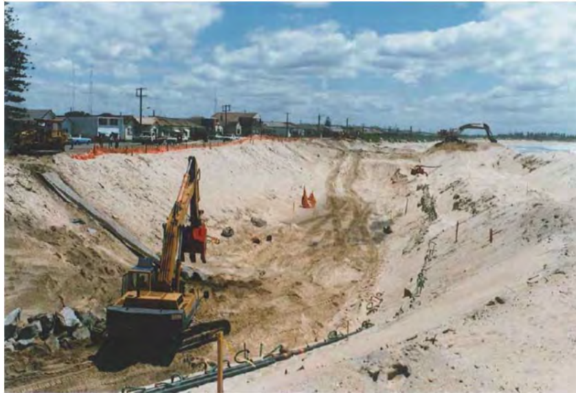
Figure 9-3 Construction of a Rock Revetment at Stockton Beach in 1987 (Photo courtesy OEH)
