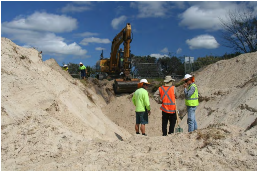
Figure 4-5 Trenching back from the beach
