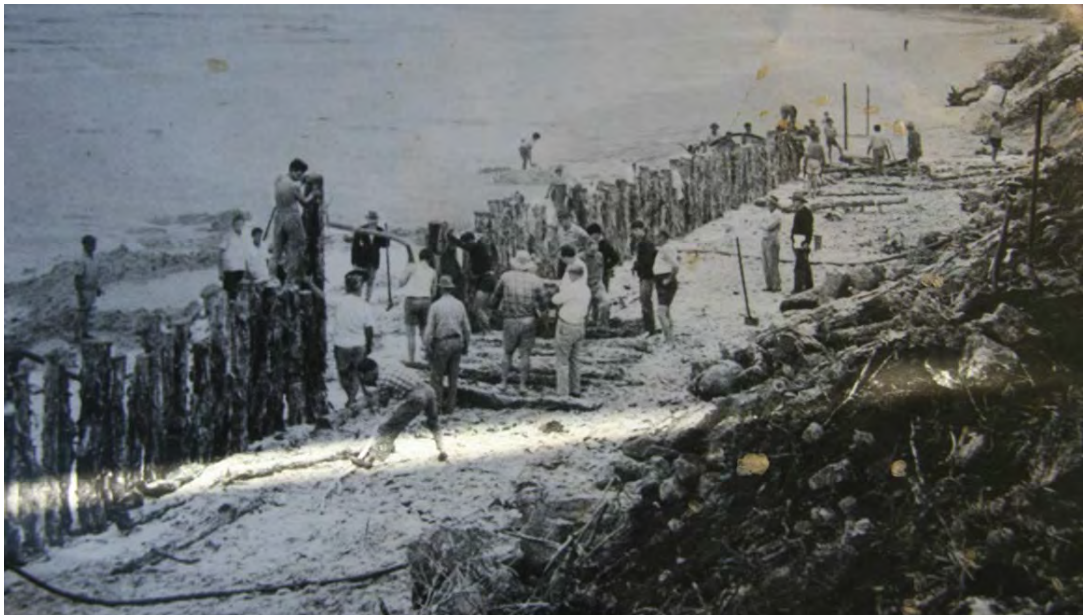
Figure 1-1 Construction of Ti-Tree Fence following 1967 Storms
