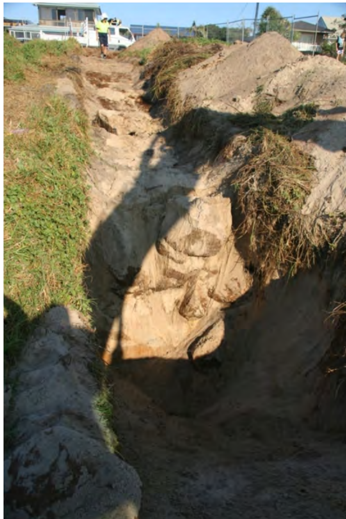
Figure 4-9 Toe of Rubble Slope
