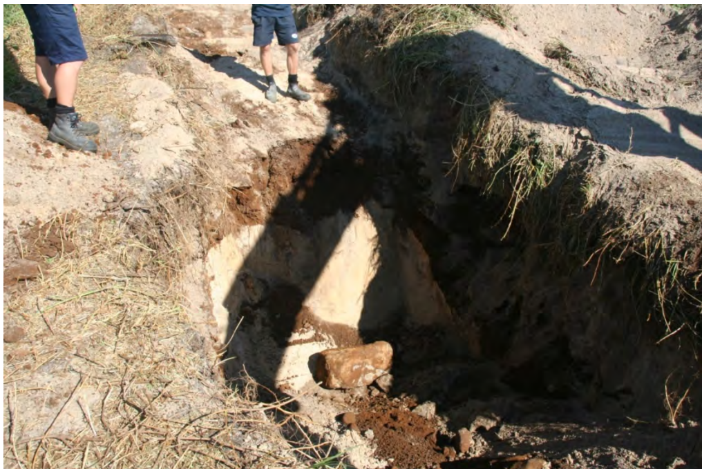
Figure 4-11 Thickness of Rubble Slope (note red soil above sand)
