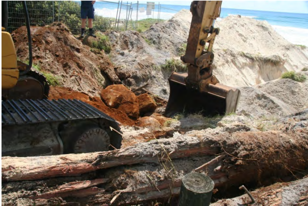
Figure 4-6 First rocks and buried power poles
