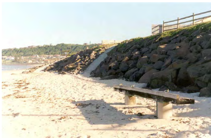
Figure 9-2 Existing Rock Revetment at Lennox Head South
