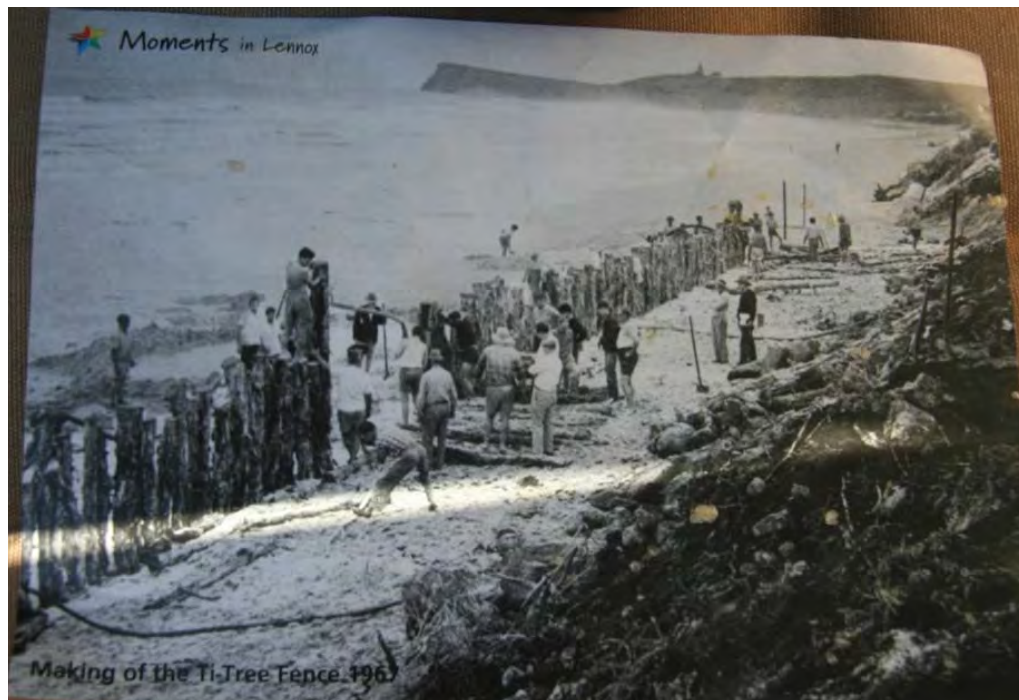
Figure 4-2 Ti-Tree Fence and rock placed on Erosion Scarp
