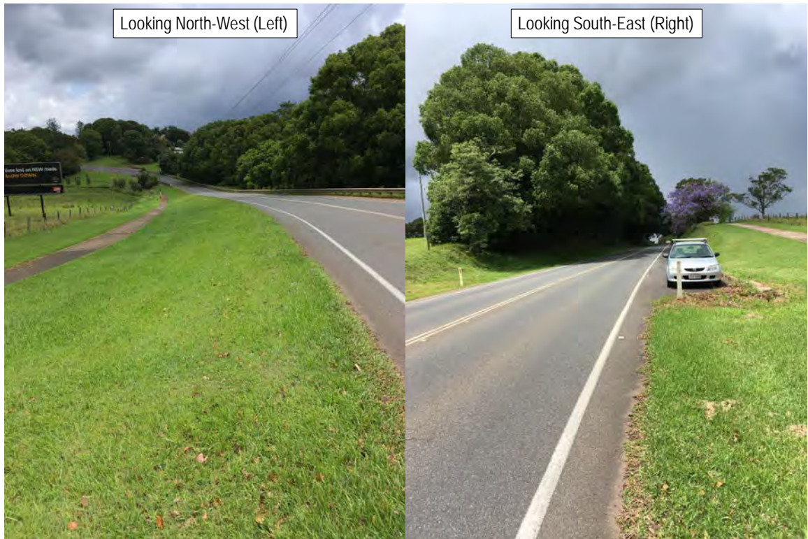
Figure 4.4: Site Visit Photos Along Lismore Road From Proposed Access Location
