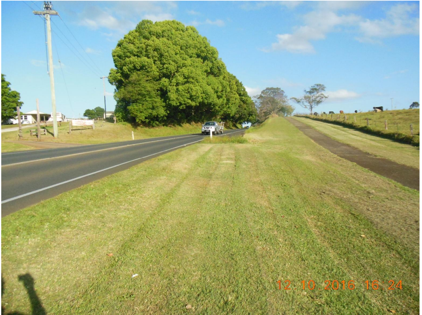
Figure 4 | Potential access location, facing east
