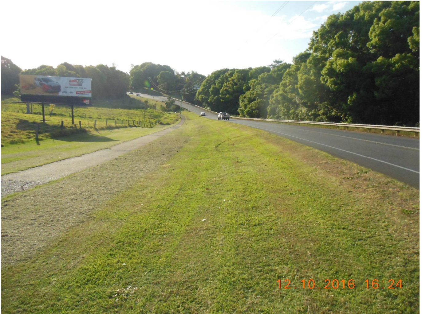
Figure 5 | Potential access location, facing west
