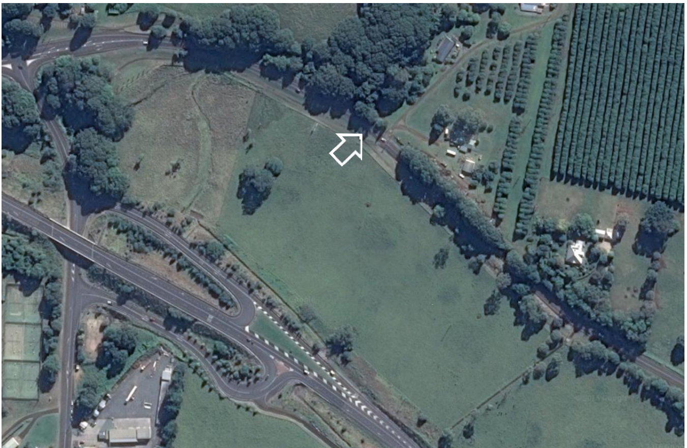
Figure 3 | Suitable access locations, Source of aerial image: Google Maps 2016
