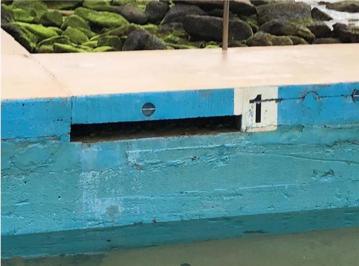
**Figure 5.1 Stainless steel lane rope attachment and scupper**
