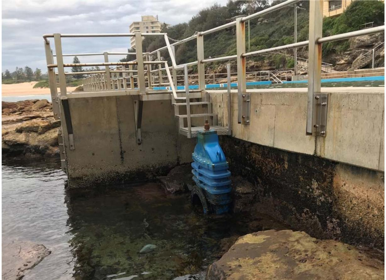
**Figure 5.6 Gate valve for draining pool**
