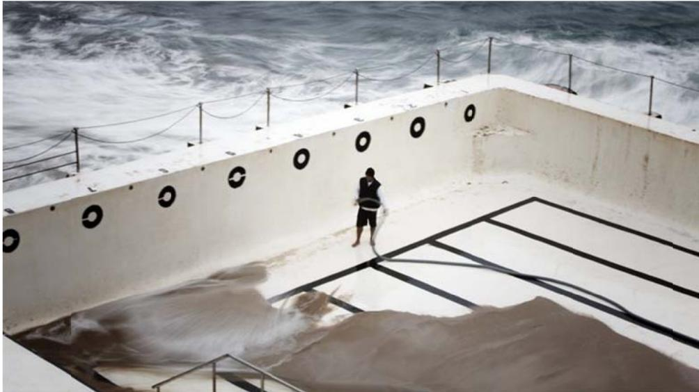
**Figure 5.8 Sand removal Bondi Icebergs (Source: Aquabumps)**
