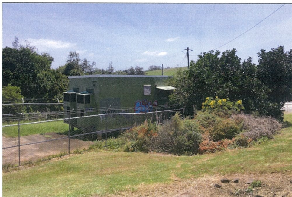
Plate 1.1: View north west from south east corner of Lot 1 showing telecommunication infrastructure.
