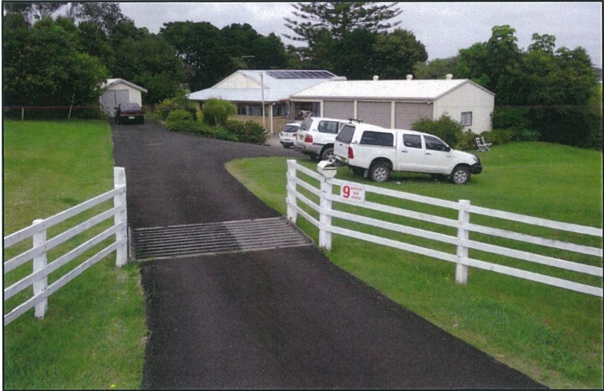
Figure 7: Lot 2 Residence precinct, view west.
