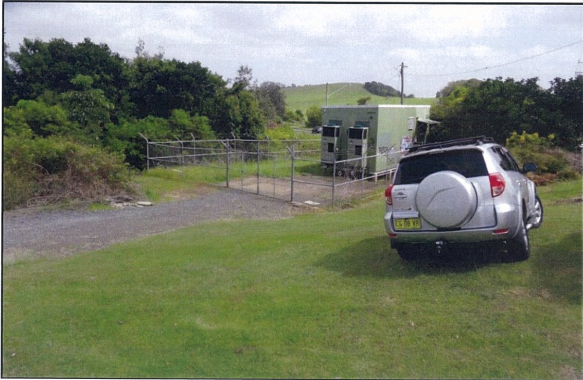
Figure 6: Lot 1 Telstra facility, view north.
