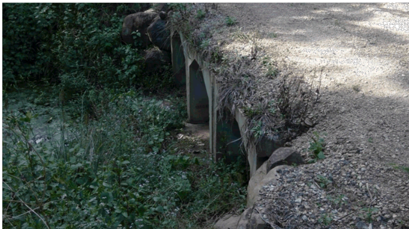
Figure 10: Concrete Culvert Water Crossing
