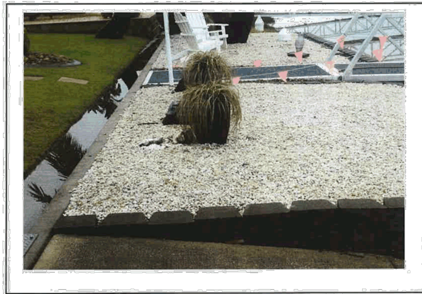
PHOTO 7 GENERAL VIEW OF COMPLETED WORKS.
