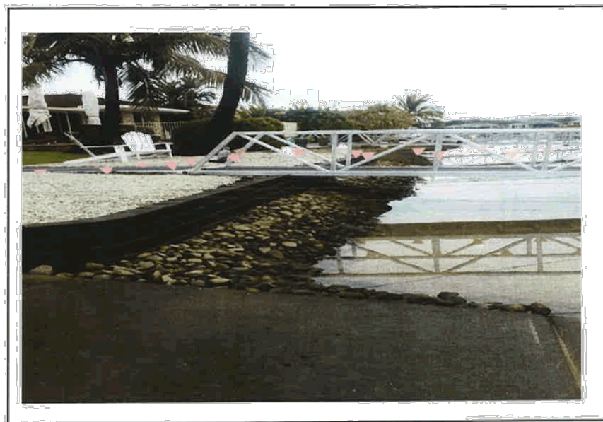
PHOTO 8 GENERAL VIEW OF COMPLETED WORKS
