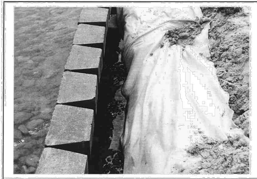
PHOTO 1 REMOVAL OF ORIGINAL WALLING AND THE DIFFICULTY IN RETAINING EXISTING BEACH DURING CONSTRUCTION OF THE REPLACEMENT WALL
