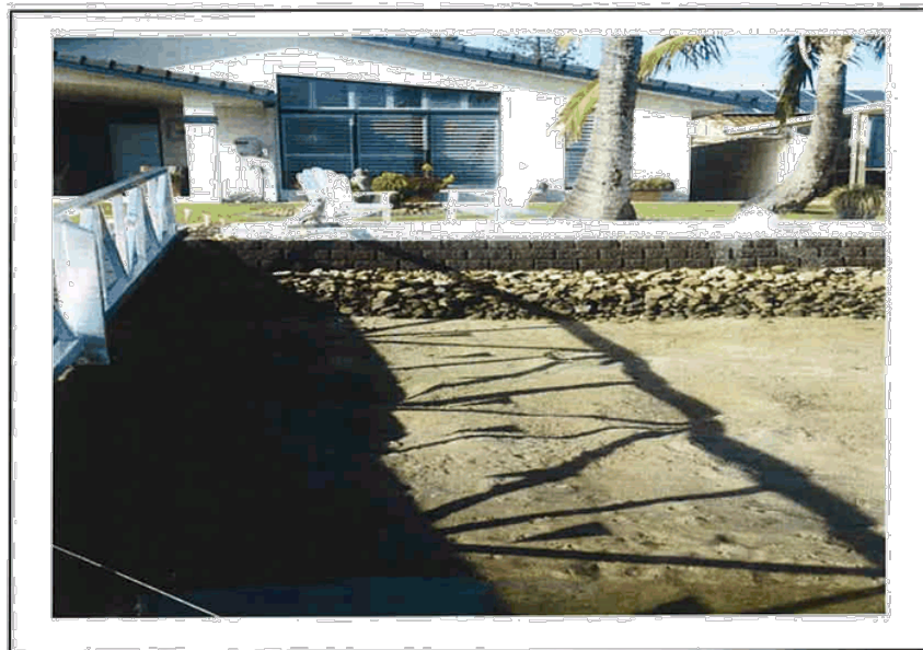
PHOTO 6 GENERAL VIEW OF FINISHED WALLING AND BEACH RESTORATION
