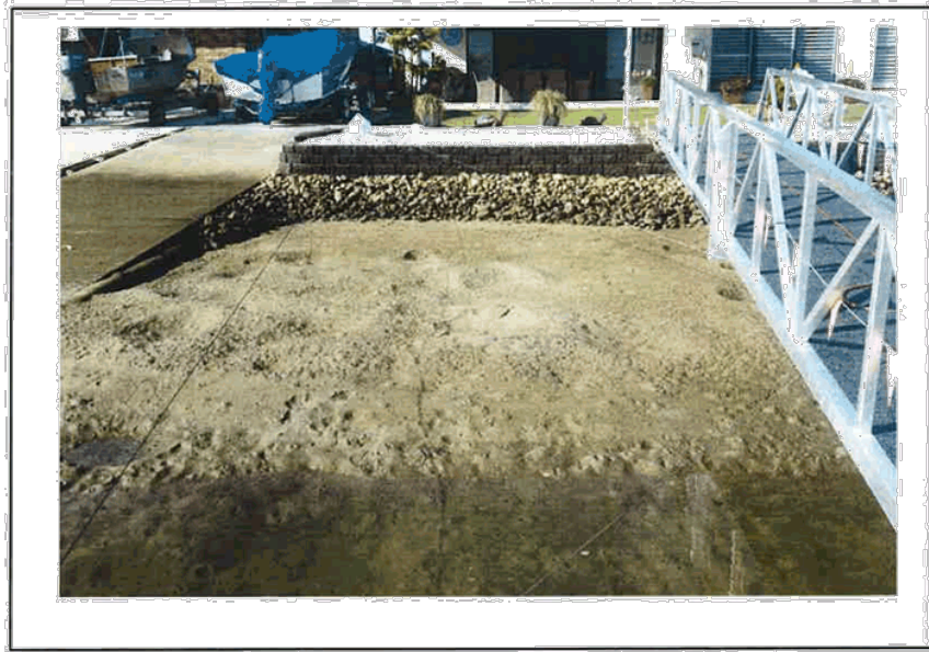
PHOTO 5 GENERAL VIEW OF FINISHED WALLING AND BEACH RESTORATION
