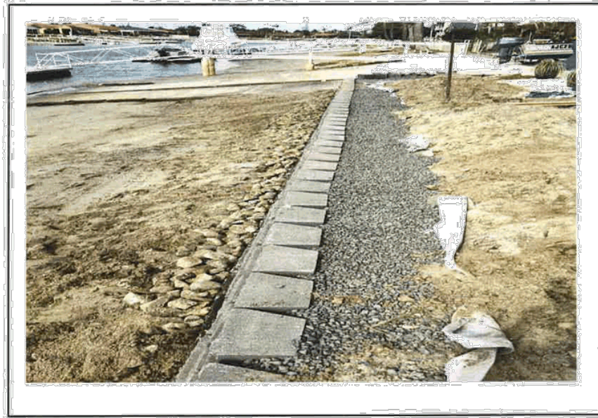
PHOTO 3 GENERAL VIEW OF REPLACEMENT WALL— BACKFILLED—NOTE EXCESS CUT BEACH MATERIAL—TO BE PLACED ONTO AND RESTORE THE BEACH.
