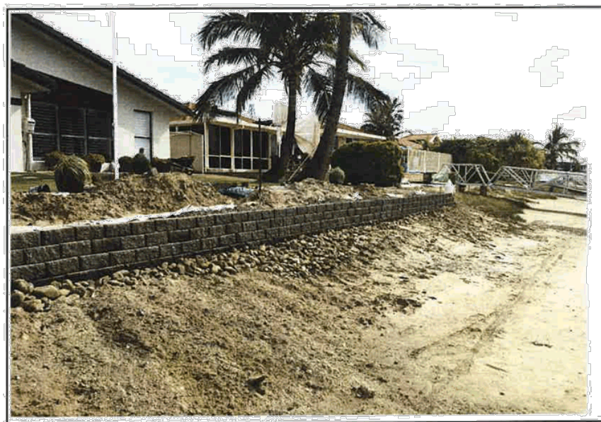
PHOTO 3 GENERAL VIEW OF REPLACEMENT WALL— BACKFILLED—NOTE EXCESS CUT BEACH MATERIAL—TO BE PLACED ONTO AND RESTORE THE BEACH.
