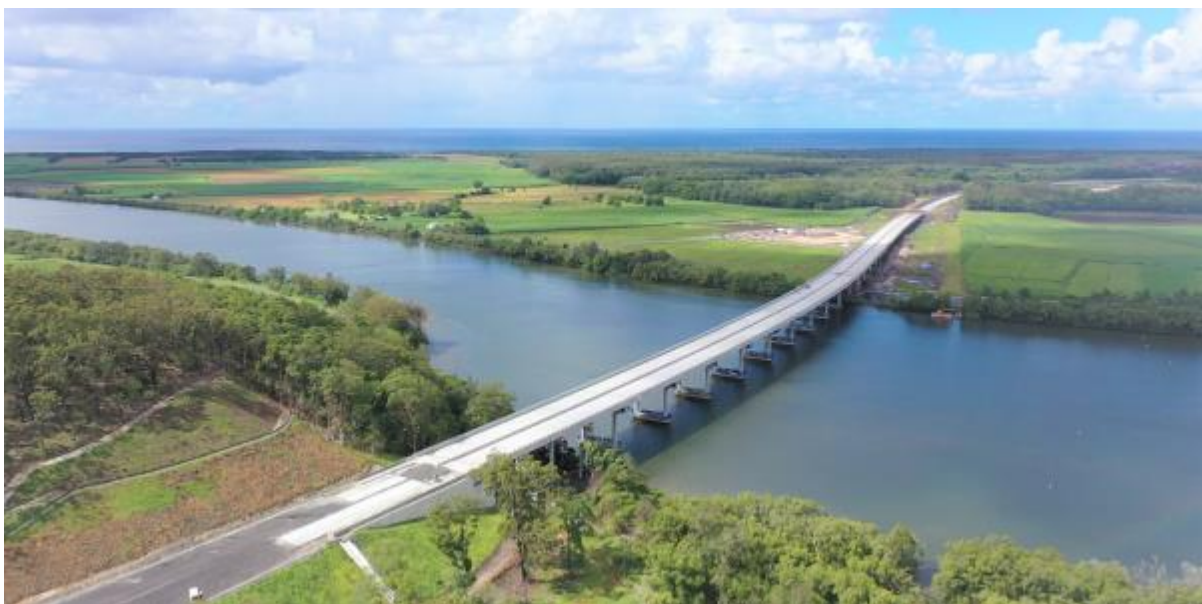
Richmond River bridge at Broadwater: Source https://www.pacifichighway.nsw.gov.au/project-sections/coffs-harbour-to-ballina/woolgoolga-to-ballina/bridge-over-the-richmond-river-at-broadwater
