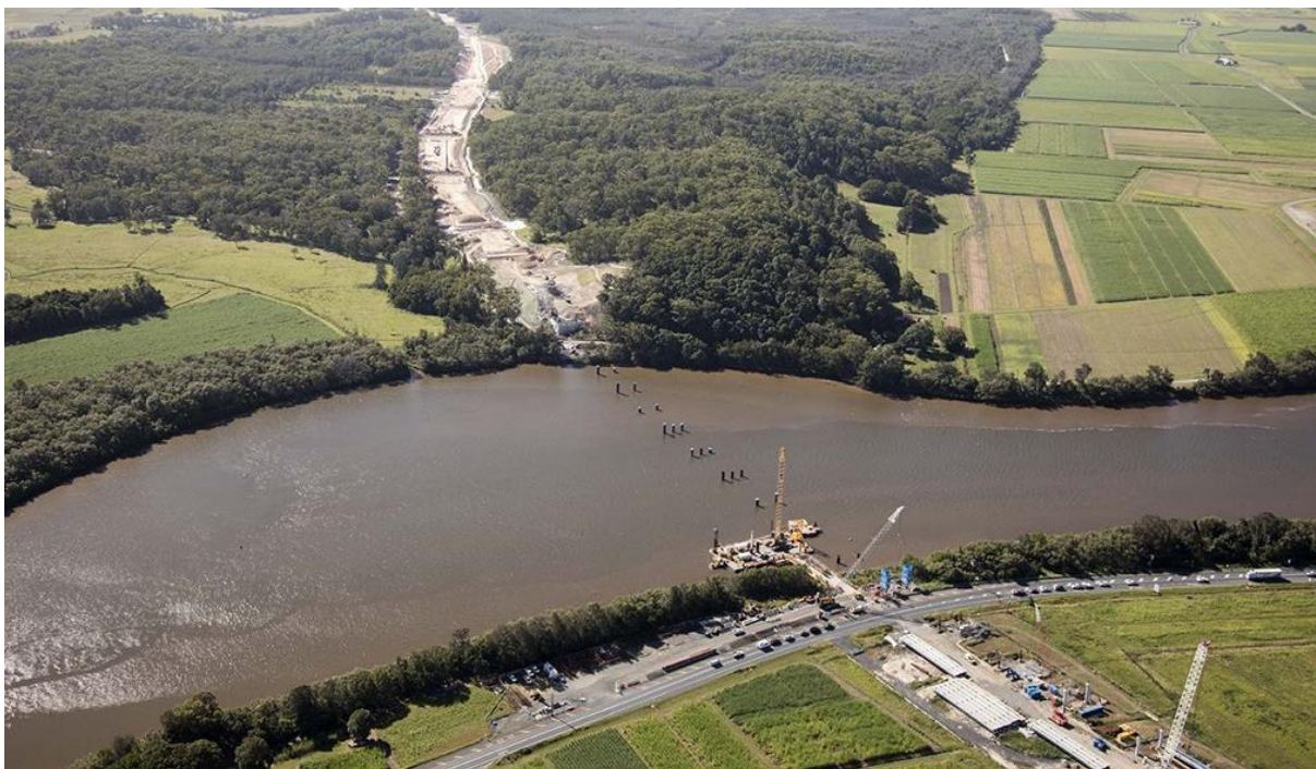
Richmond River bridge construction at Broadwater: Source https://www.pacifichighway.nsw.gov.au/project-sections/coffs-harbour-to-ballina/woolgoolga-to-ballina/bridge-over-the-richmond-river-at-broadwater
