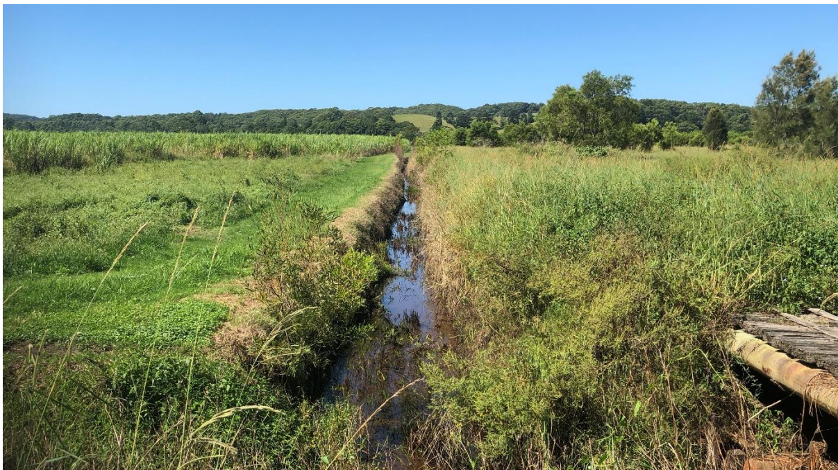
North Creek – linear drain in upper catchment (2018)
