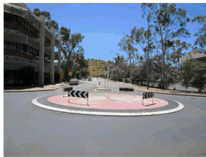
Completed Roundabout- Alice Springs
